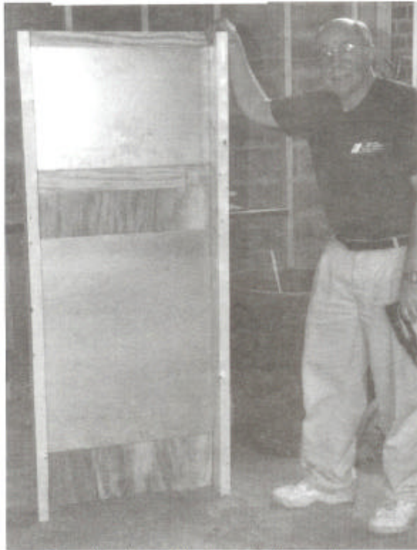
Completed stands before installing cardboard.
